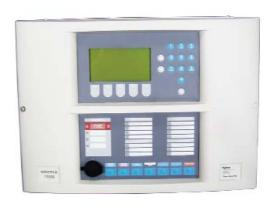
The decision to sound the alarm is made at the controller allowing adjustments and compensations to be made for changes in environmental conditions. In short, maximum security whilst minimising the risk of false alarms.
