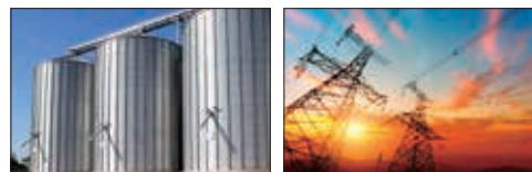
Hazardous Storage Tanks Transmission Towers
